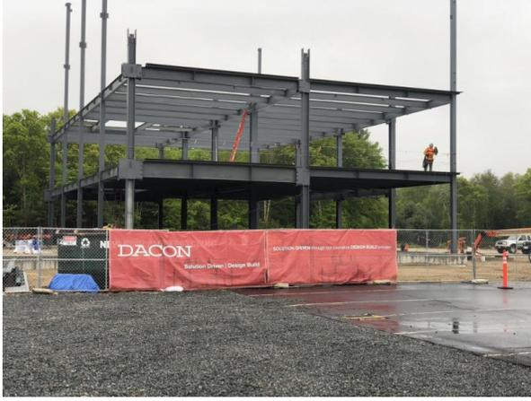
one day and the Engineer of Record, RRC Engineering was impressed enough to move our design right into motion. The schedule required really fast movement and with SidePlate field-bolted connections, things did happen quickly. Within four weeks of starting to assemble the steel frame, Dacon Corporation, the General Contractor, Norgate Metal, the Steel Fabricator, and Brouchard Steel Erectors, the Erector, were thrilled with their first SidePlate project.
